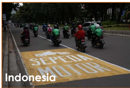
Jl. MH Thamrin and Jl. Medan Merdeka Barat, Jakarta, Indonesia extensão = 5km largura = 3.0m - 5.0m
